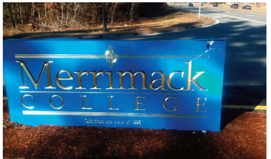
Damage was reported on Sunday January 29 to the 125 entrance sign. According to Police Services there is no information as to what caused the damage.
