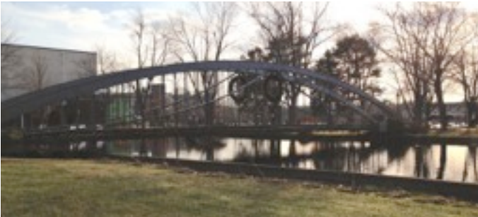
Moseley Wrought Iron Arch Bridge on a December afternoon.
