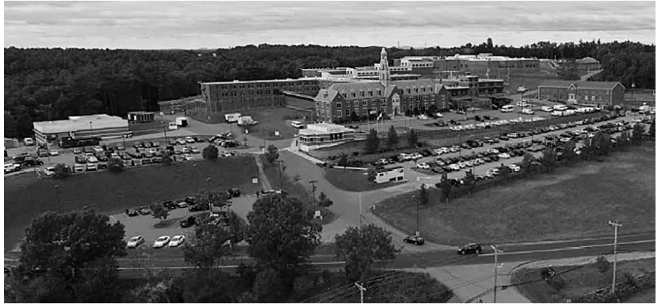
The Essex County Correctional Facility, in Middleton, Massachusetts.
