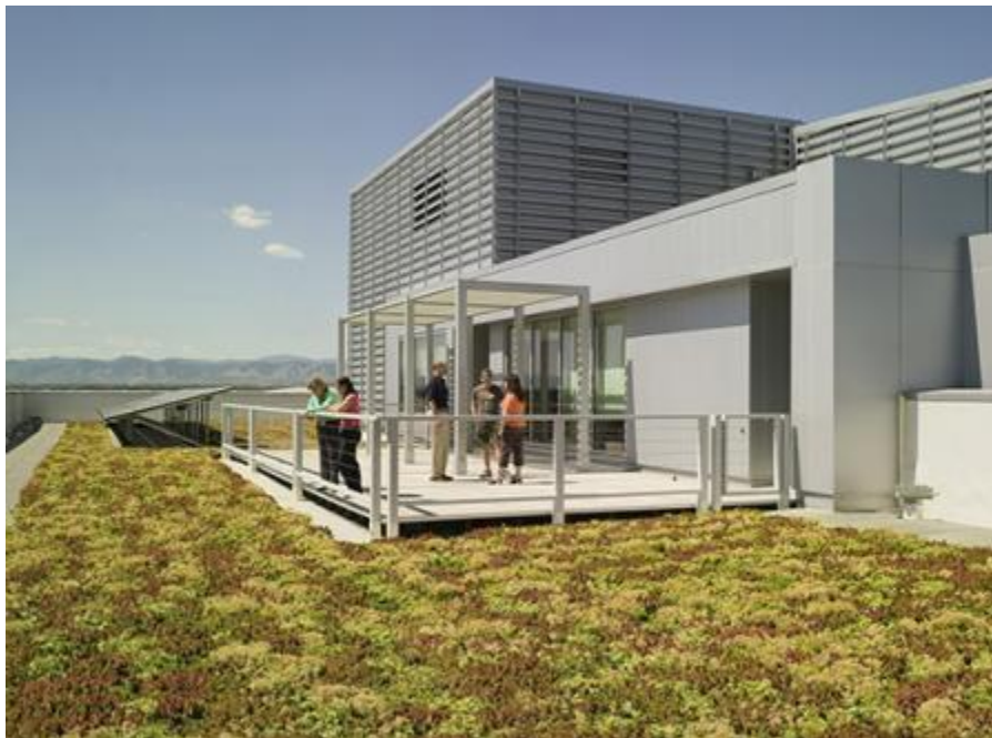
Figure 1: Pictorial Representation of EPA Region 8 Headquarters Green Roof (EPA, 2019).
